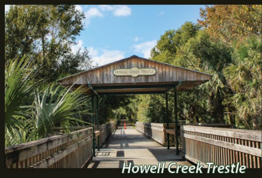
Howell Creek Trestle
