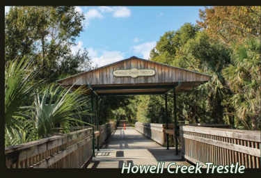
Howell Creek Trestle
