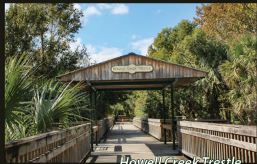
Howell Creek Trestle
